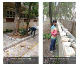
Tree grates and leveling the Rajakaluve SWM wall
